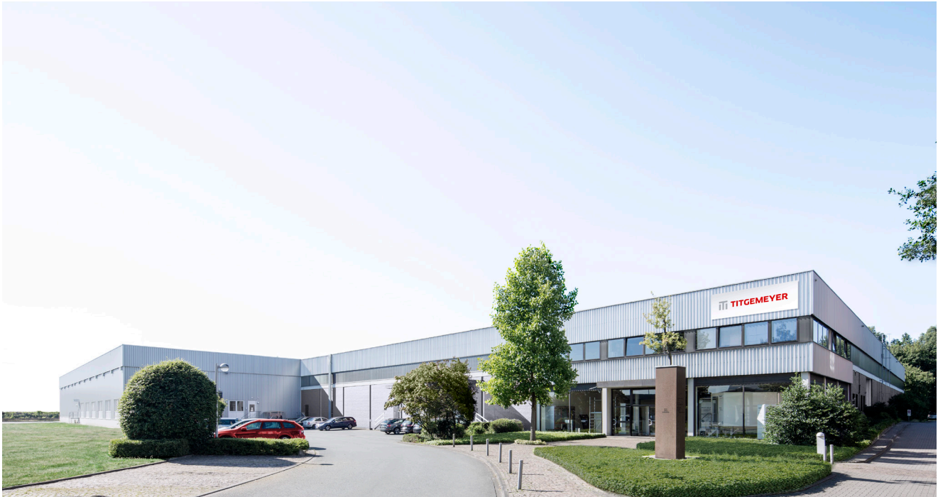
Central warehouse in Osnabrück
